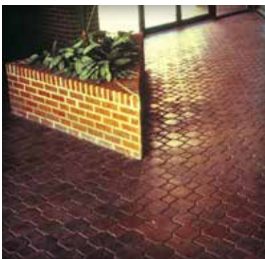
Figure 1. Many sealers enhance the appearance of concrete pavers and protect against staining.
