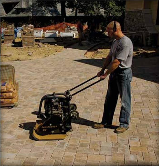
Figure 9. Compacting the pavers and bedding sand.
