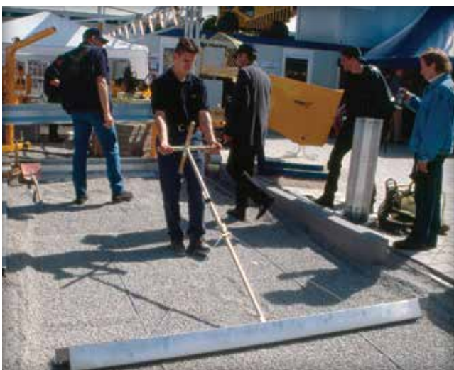
Figure 25. Manually screeding the No. 8 stone setting bed.
