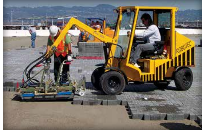
Figure 4. Hydraulic clamp picking up layer of pavers
