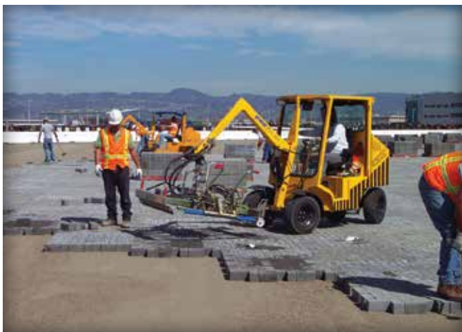
Figure 5. Motorized equipment with a hydraulic clamp.
