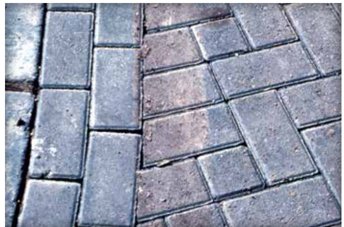
Figure 14. A double row of manually placed pavers along a curb or building provides maneuvering space for the mechanical installation clamp.
