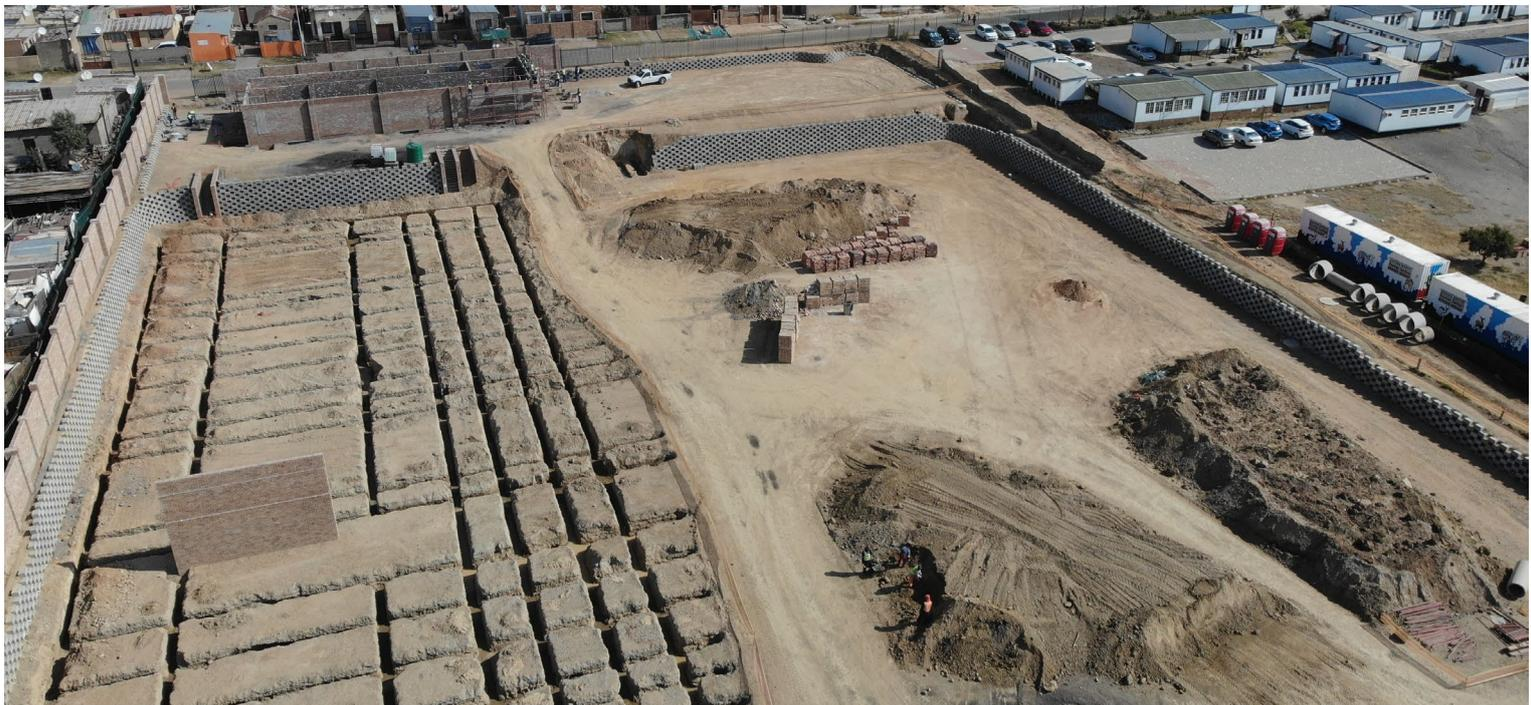
A no-fines concrete mix requires a specified mix-design - eliminating fine material sand from the mix, that once hardened, has a higher permeability than standard concrete mix-designs. For CBR walls this is an advantage because the no-fines concrete allows any water seepage to permeate through the concrete and can then be captured by weep holes situated at the base of the wall.
