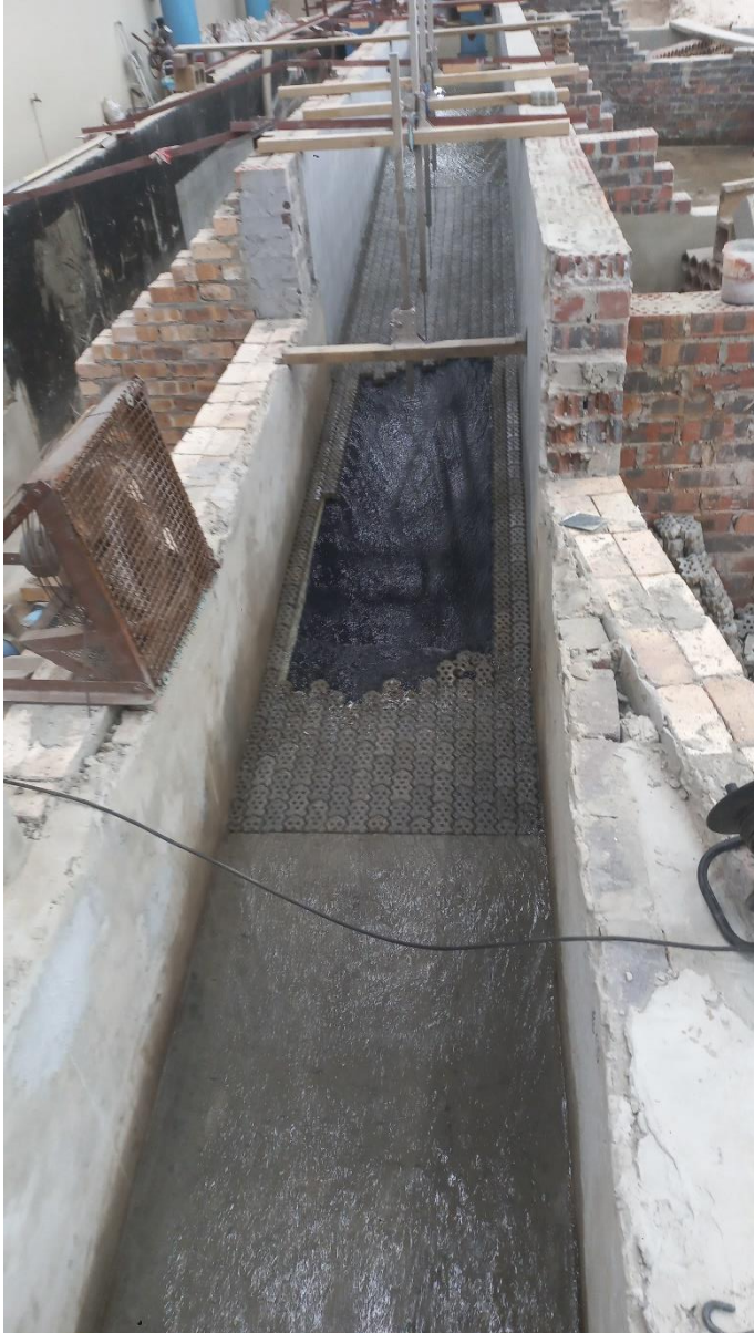
Figure 3-4: Photograph of the test blocks after failure at 160 L/s for the 1:10 slope longitudinal bed slope
